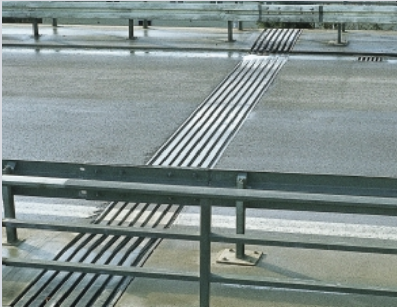
Girder Grid Joint type D 560
