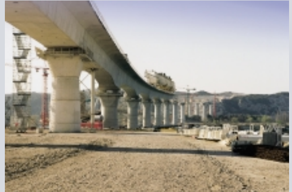
TGV Viaduct, Avignon
