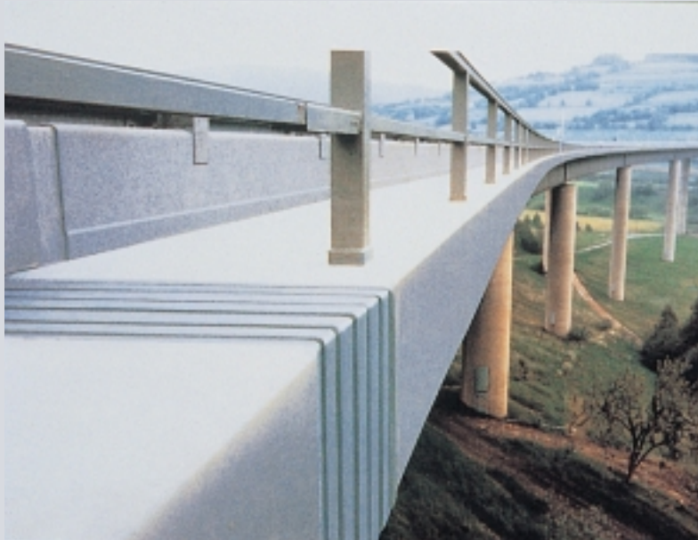
Watertight design of parapet
